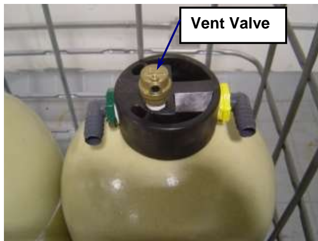
Figure 6: Filter Air Vent Valve
